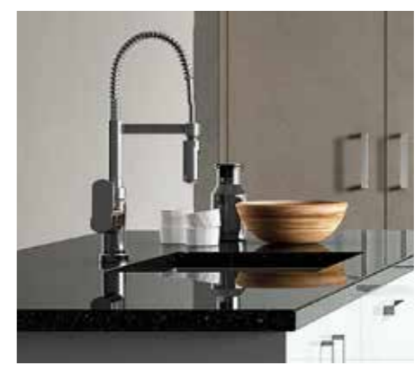
Undermount sinks help create a flow to the kitchen and add a touch of class.
